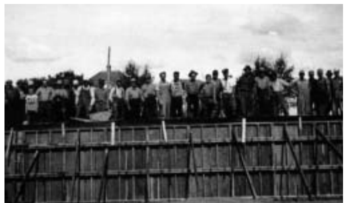
Work Crew on Perdue Legion Hall 1952
