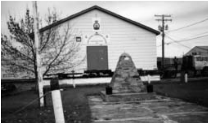
Spiritwood Legion Hall moving on to new foundation.
